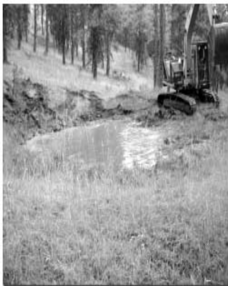
Swamp Creek Habitat Improvement Project
