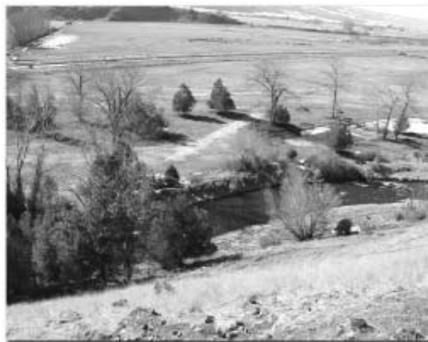
Project Area Pre-Excavation Photo Taken March 9th, 2004
